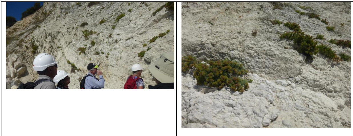
This cliff face is a major fault. Slickensides are very visible
